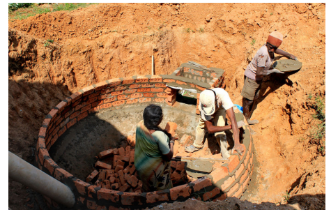
Beneficiaries constructing the digester with help of bricklayers of SKG.
